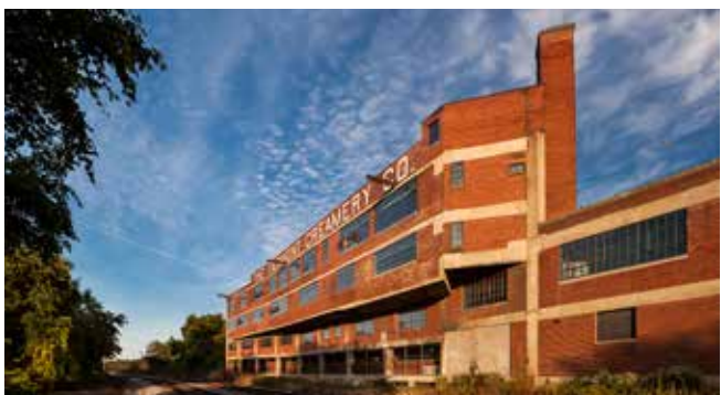
Image: Courtesy of Christian Phillips Photography A look at the exterior of The Fairmont Creamery in Cleveland, a former creamery that Sustainable Community Associates used historic tax credits (HTCs) to develop into a 30-apartment building.
